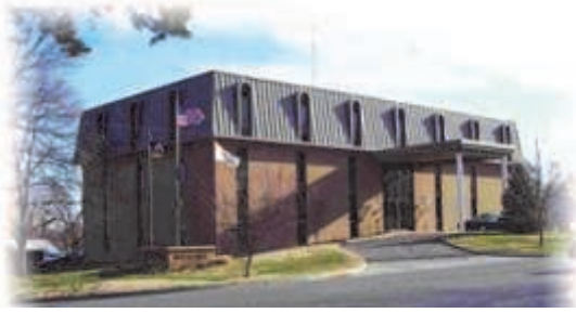
Roeland Park City Hall 1995-current
