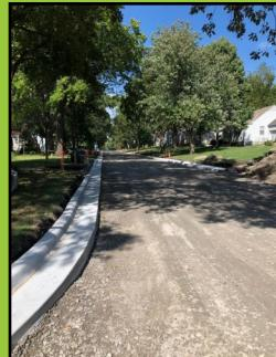
Construction on Rosewood is nearing completion. Expect the street to be fully functional by the end of October. Rosewood from 55th to Alder was part of the Residential Street Reconstruction program and will include new curbs, gutters, resurface, minor storm sewer repairs and a new sidewalk.
