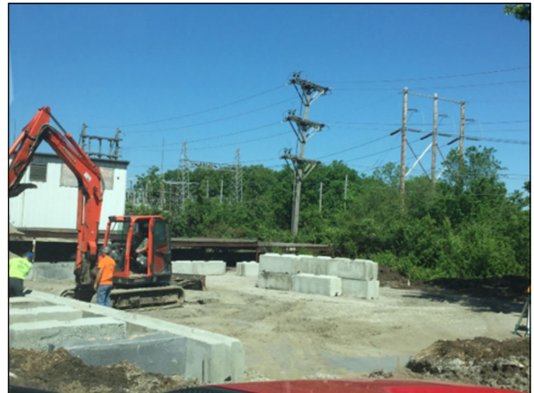
Base of the Dome being laid and the concrete blocks being placed prior to concrete floor.
