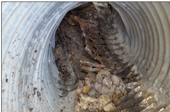
Condition of Existing Pipe showing rust
