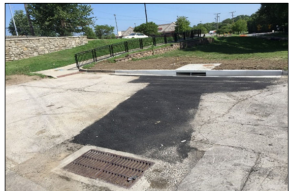
Restoration of Granada Street with new inlet
