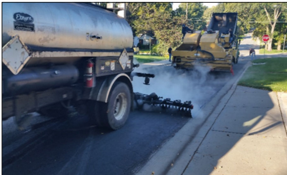
Oil Sprayed on Streets for Granite Chips
