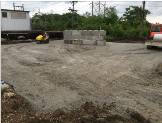
Base of the Dome being laid and the concrete blocks being placed prior to concrete floor.
