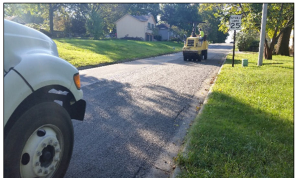
Granite Chips (Rock) Placed on Oil, Then Rolled
