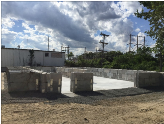
The Concrete Block Walls installed and the Concrete Floor has been poured with separation wall.
