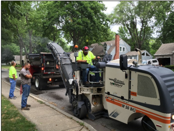
Public Works Removing Bad Asphalt
