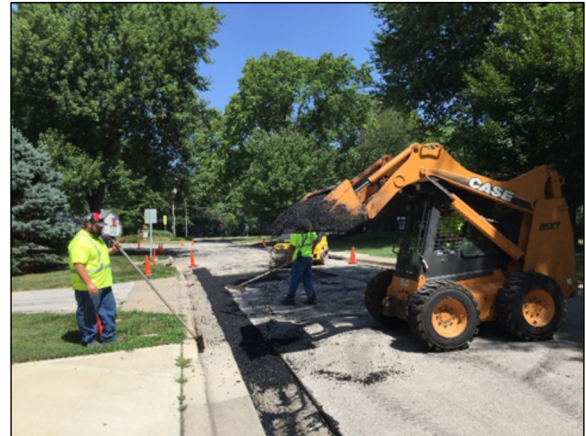
Public Works Placing New Asphalt
