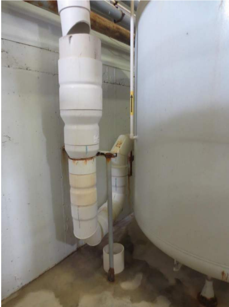
Filter Backwash Discharge
