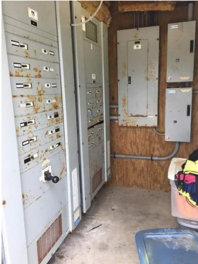
Electrical Control Room (note corrosion)
