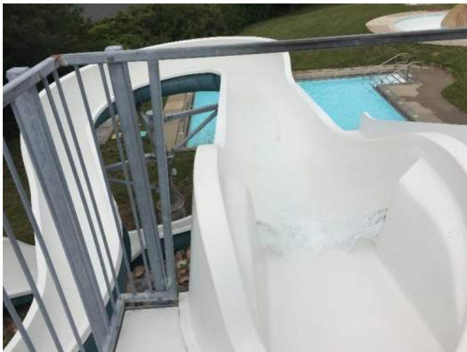
Water Slide Entry Tub (Challenges Visibility to Plunge Pool)
