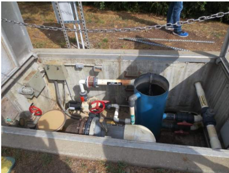
Flow Control Pit for Water Slides
