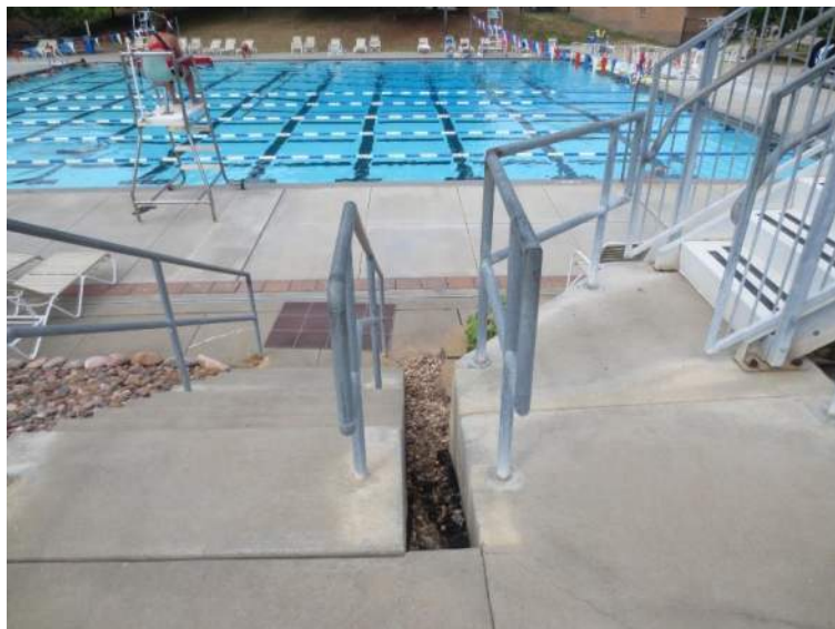
Slide Handrail Gap
