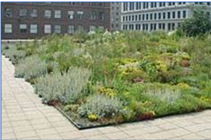
Green roofs are one technique that helps reduce heat island effects, lower energy consumption, and manage storm water runoff.
