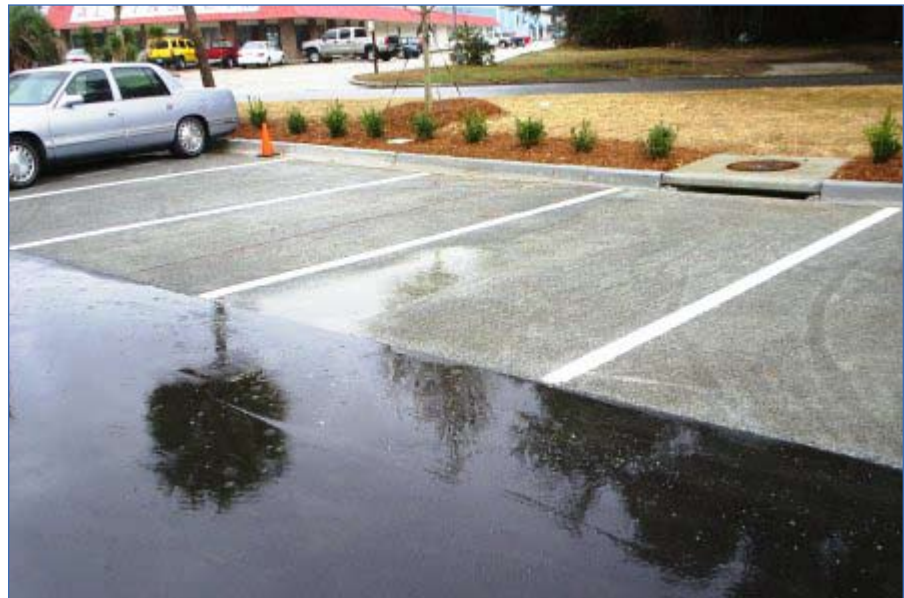
The use of pervious paving materials let air and water pass through, filtering pollutants on the spot and reducing the 'heat-island' effect of traditional asphalt and concrete paving. Options include porous aggregate, open-jointed blocks, pervious concrete and porous asphalt.
