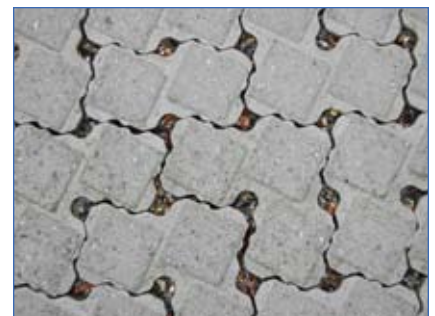
Pervious pavers provide a hard, reliable walking and driving surface, while still allowing 100% rainwater infiltration.
