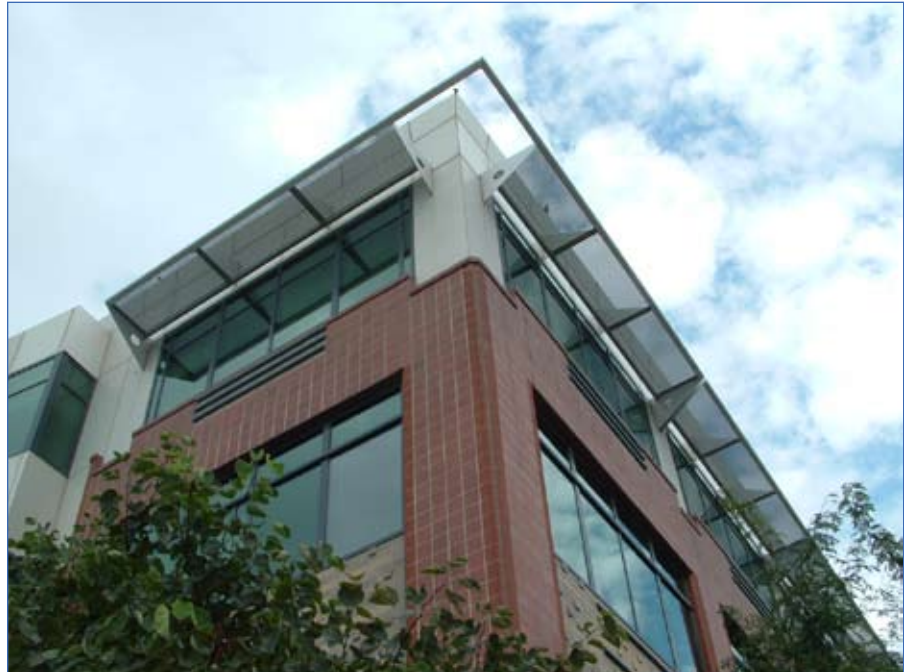
The appropriate use of exterior shading devices and glazing parameters can directly reduce heat gain and loss of the building, and are potential technologies and strategies for LEED certification.
