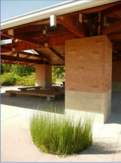
Filtration areas below downspouts help reduce stormwater runoff and improve water quality.
