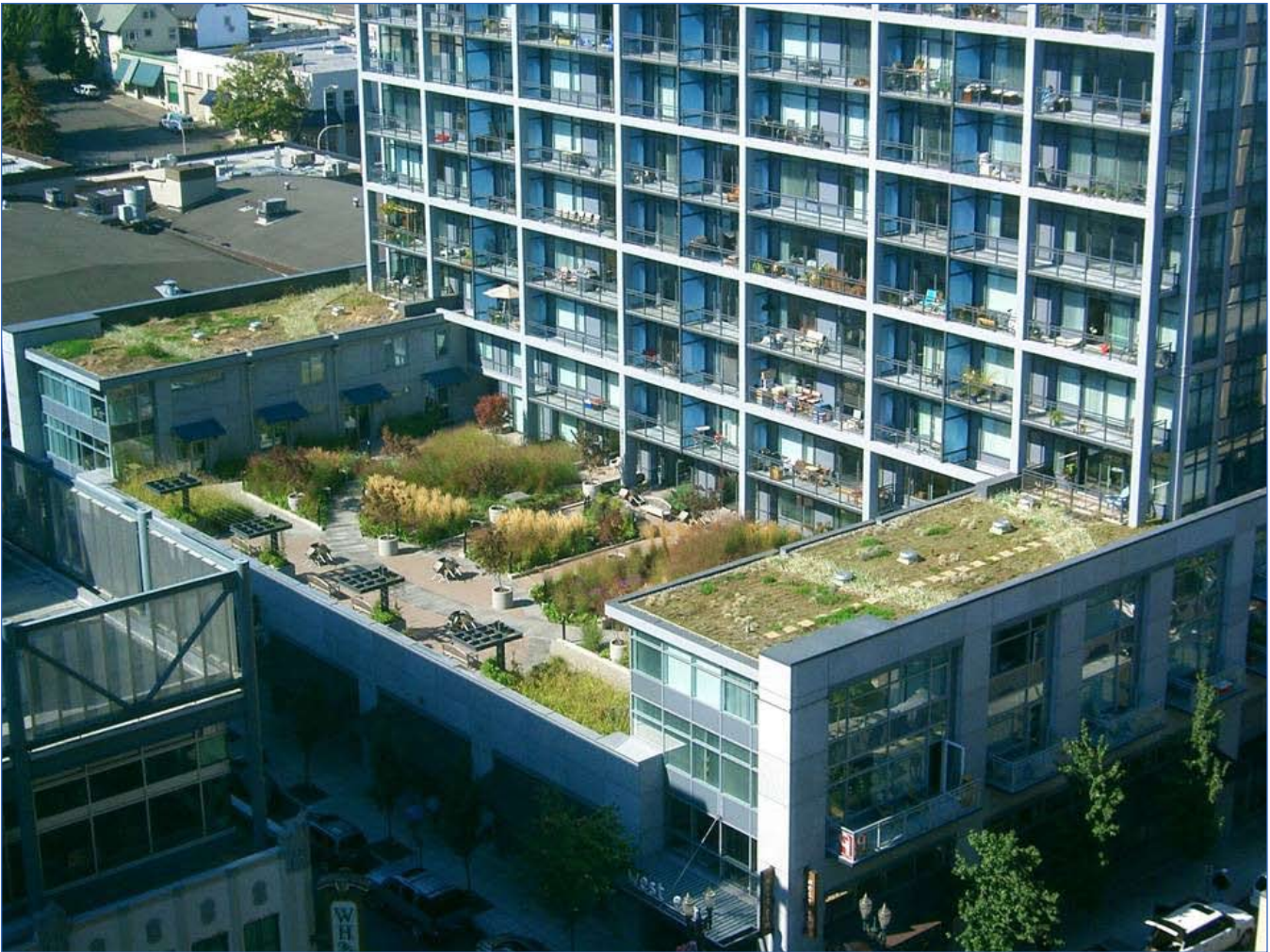
Green roofs can provide amenities for building occupants, as well as enhance site sustainability by reducing heat islands and managing storm water runoff.
