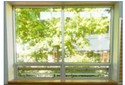
The use of operable windows made of low-emission glass should be considered as a means of increasing ventilation through the building and reduces heat gain.
