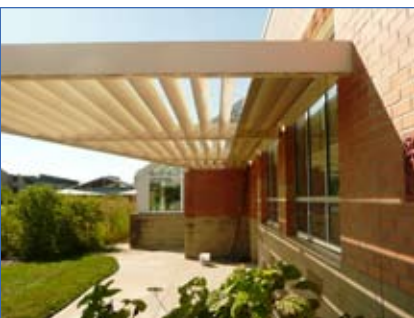
The width of an overhang should be carefully calculated for the most advantageous degree of solar control.
