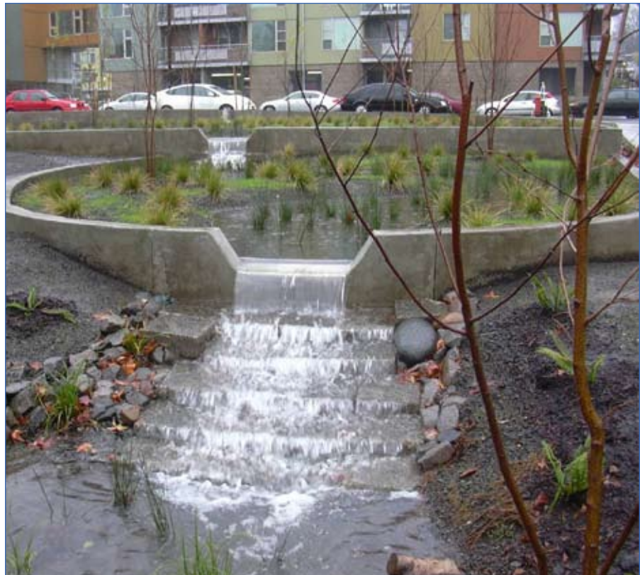
Constructed rain gardens can help alleviate stormwater runoff, improve water quality, and add to the landscaping design of a public park or plaza.
