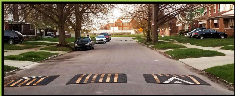
Example of a temporary speed hump with wheel cutouts for emergency vehicles.
